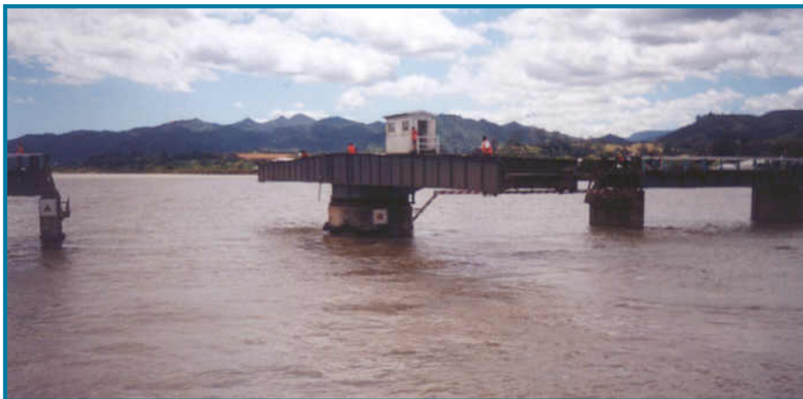
The Kopu Bridge
